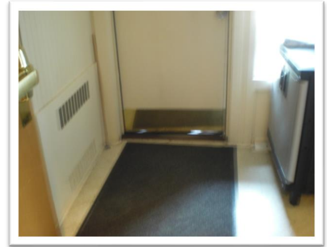
Gaps under doorways
