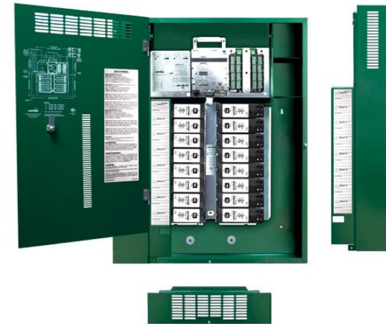
Lighting control panel
