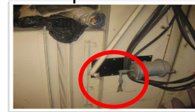
Disconnected Damper
