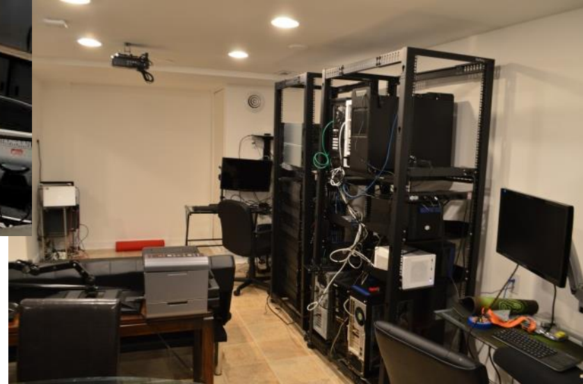
Server Rooms Served by Central HVAC
