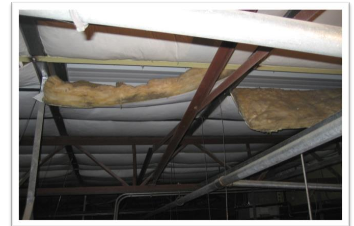
Failed roof insulation
